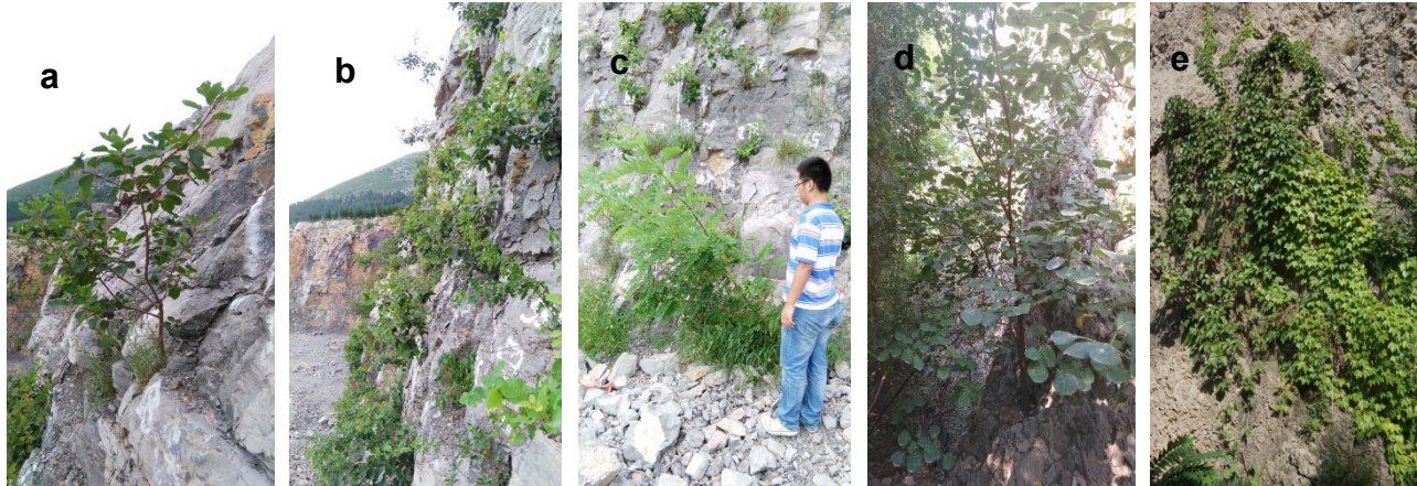
Figure 8 Growth of revegetation plants on the high and steep rocky slope in 2019. (a) C. coggygia var. cinereus Engl.; (b) Side view of slope; (c) R. pseudoacacia Linn.; (d) C. coggygia var. cinereus Engl.; (e) P. tricuspidata (Siebold & Zucc.) Planch.
