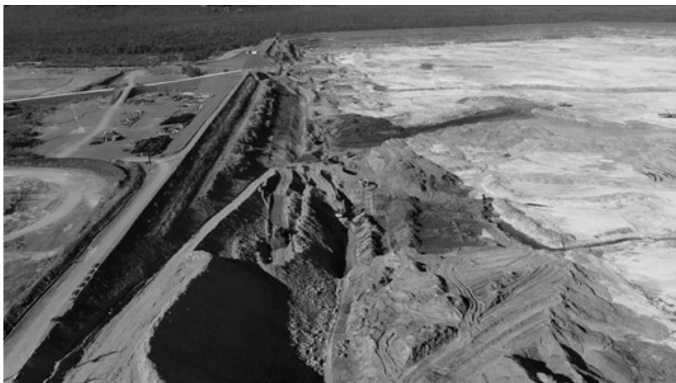
Figure 6 Image from drone flyover, showing north-east ramp construction in May 2021
