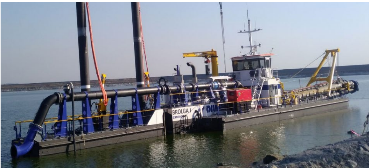
Figure 3 TSF dredging operations with Jabiru and Brolga I cutter suction dredges
