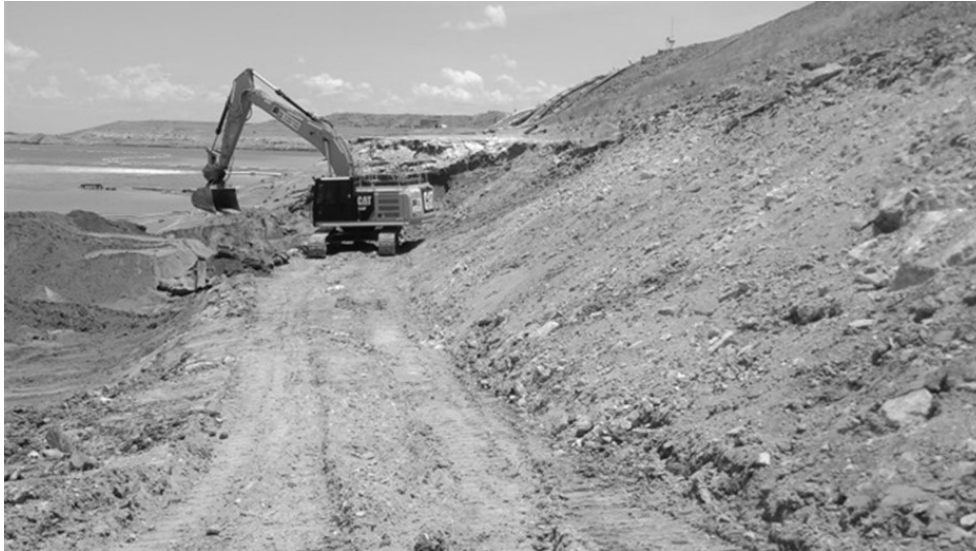
Figure 5 Excavator on temporary working platform inside the dam during dredging operations
