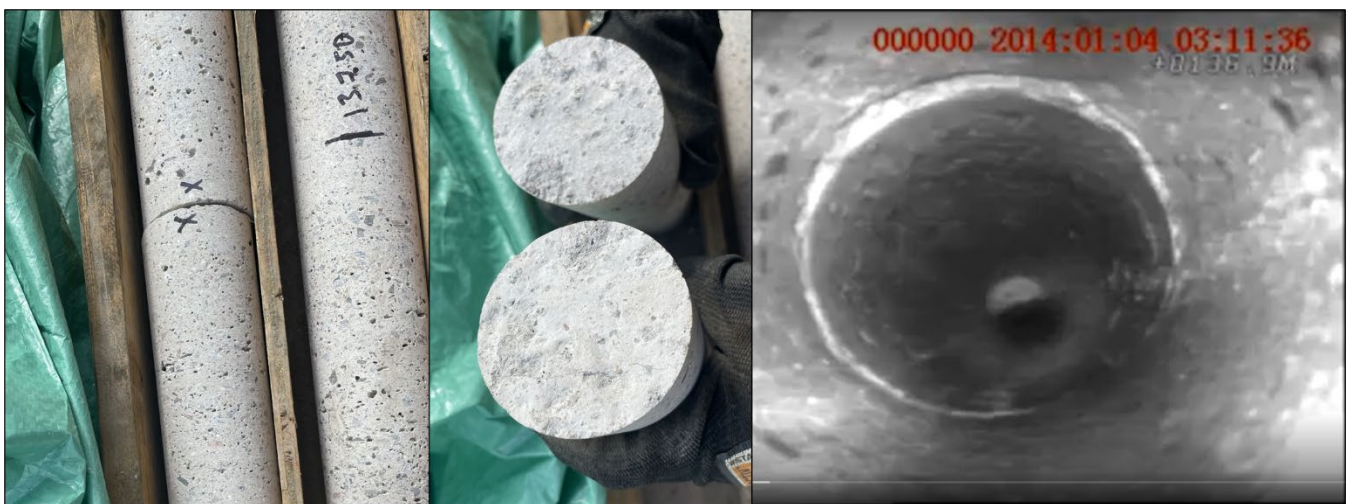
Figure 9 Interpretation cold joint in box (left), split to expose surfaces (centre) and in borehole camera video (right) from borehole 4 at 136.9 m along hole/28.01 mamsl
