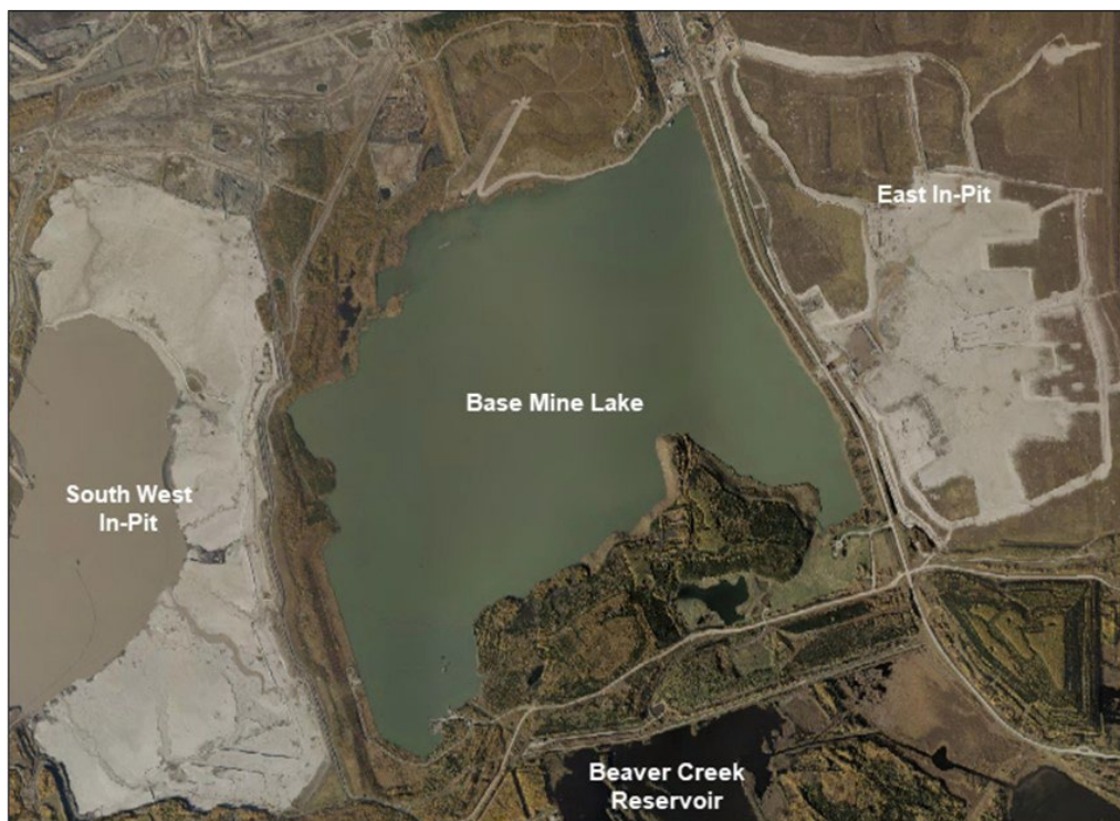
Figure 1 BML showing adjacent structures and Beaver Creek Reservoir (BCR)
