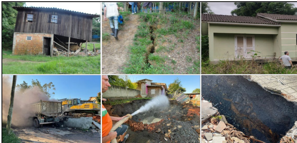
Figure 8 Houses with subsidence caused by underground mine workings within the urban area of the municipality of Criciúma, and houses built over tailings affected by spontaneous combustion.
