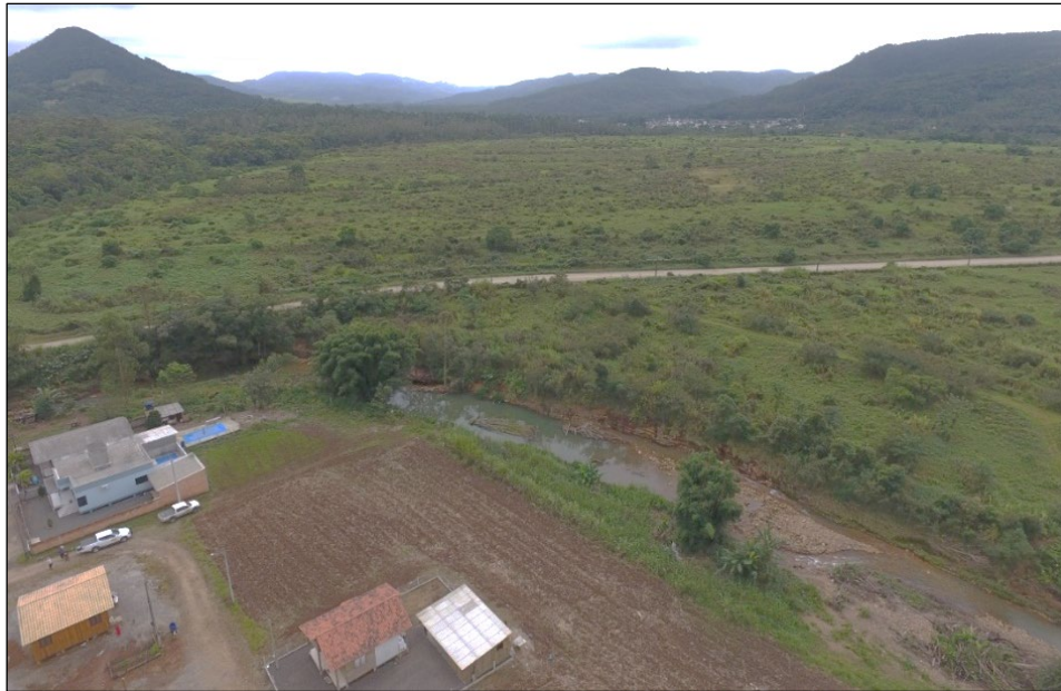
Figure 10 Image of the rehabilitated area where it is possible to observe the presence of tree and shrub species that may have penetrated the 50 cm layer of compacted clay that isolates the tailings.
