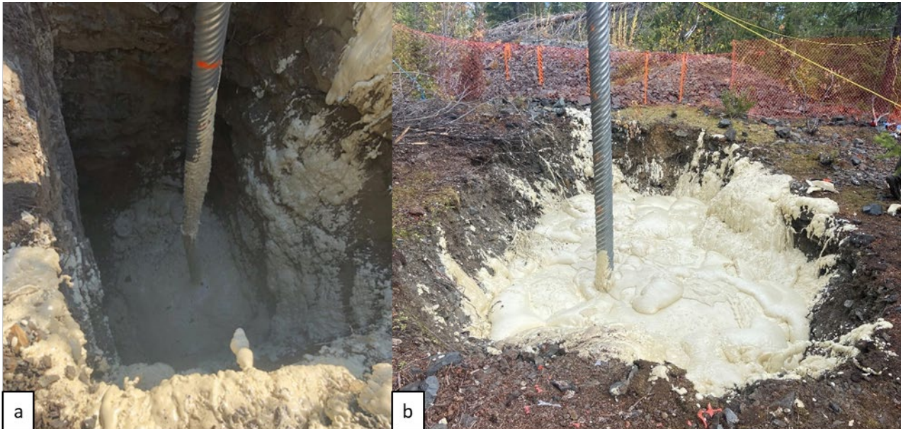
Figure 3 (a) Lift 1 following placement (b) Lift 17 following placement
