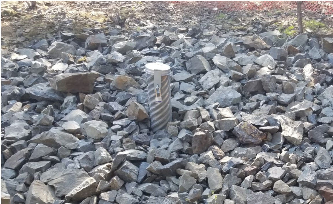
Figure 4 Completed polyurethane foam plug
