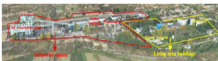
Figure 2 UAV aerial panorama
