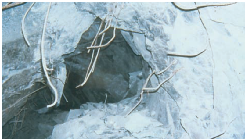
Figure 3 Complex loading of rock reinforcement elements captured by WD Ortlepp (Stacey 2012)
