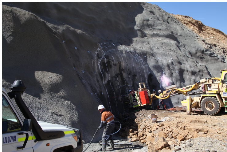
Figure 12 Bench face and portal mark-up prior to the commencement of blasting
