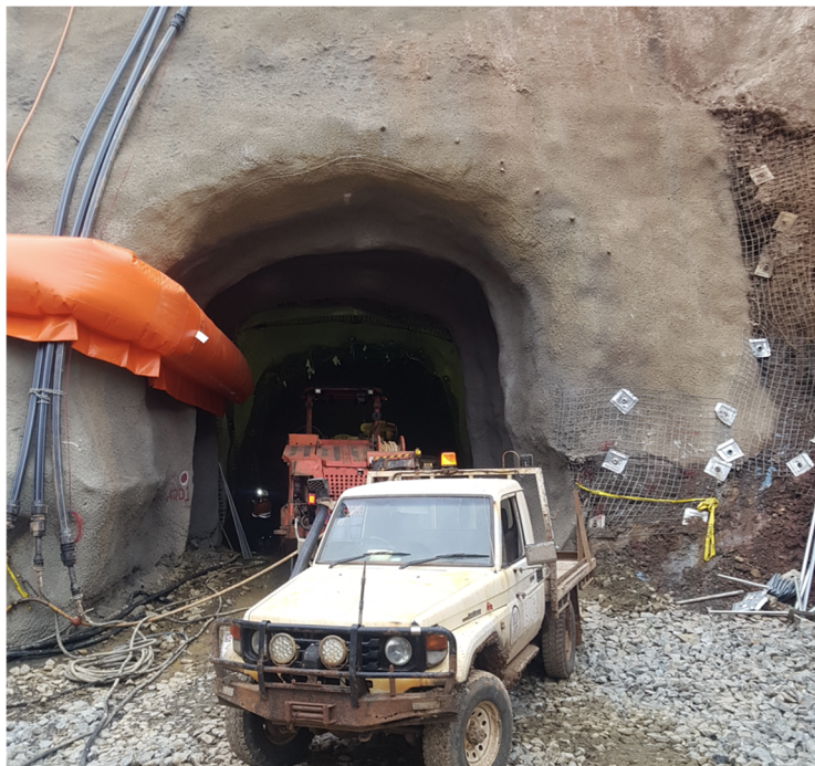
Figure 5 Portal development commenced and \approx 20 m long
