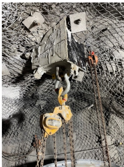
Figure 8 Lifting base for liner installation, Andes Norte, El Teniente
