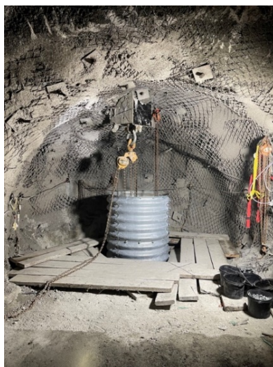
Figure 9 Steel liner column installation process, Andes Norte, El Teniente
