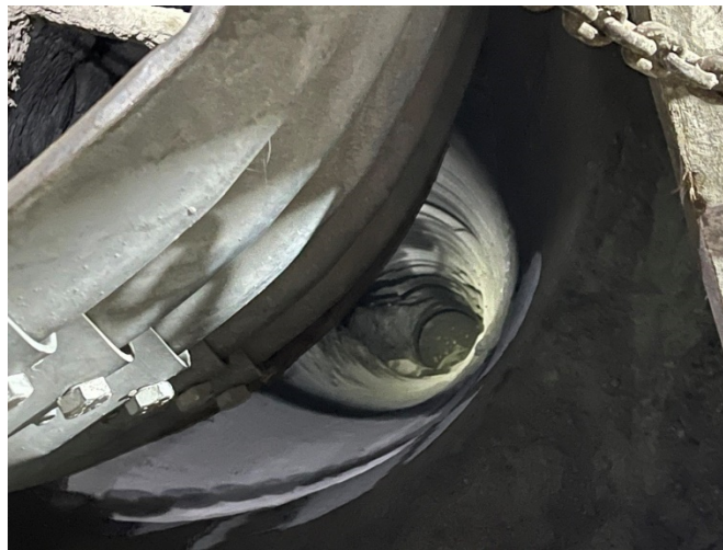
Figure 4 Picture of a post-excavated shaft, Andes Norte, El Teniente (Codelco 2023)
