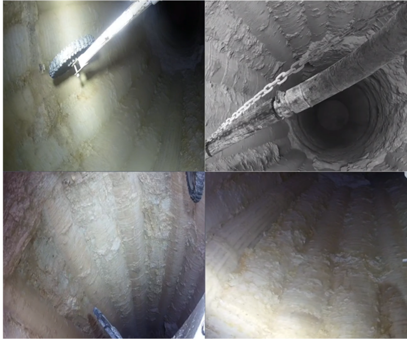
Figure 3 Example of exposed secant piles after raiseboring
