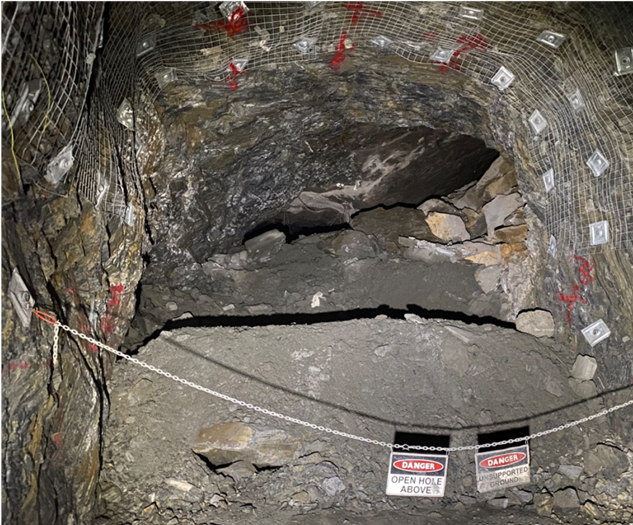
Figure 4 Large-scale cavity at the scale of an underground development drive
