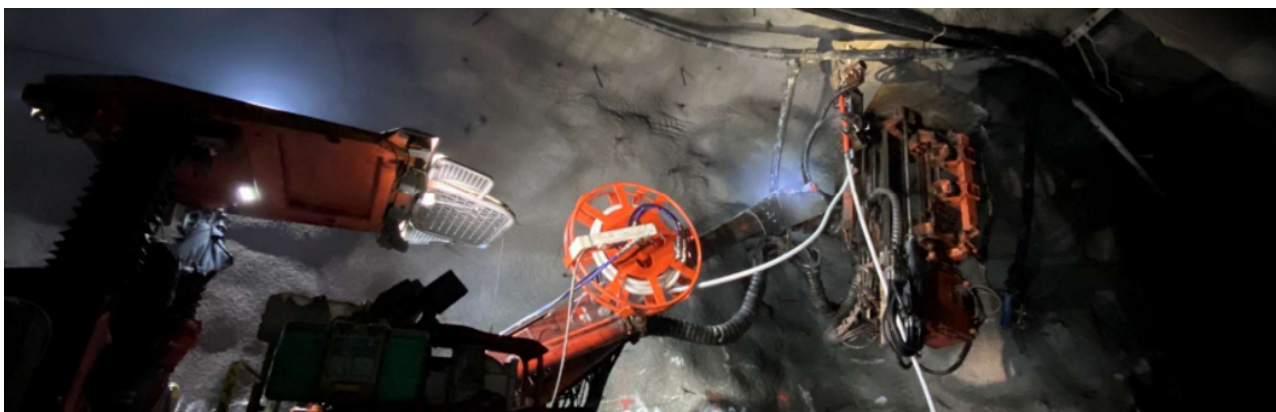
Figure 23 J-Lok P resin injection utilising a standard Sandvik grouting process
