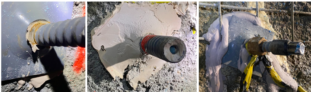
Figure 7 Polyethylene-coated dynamic MPA and Falcon Bolts installed and grouted with polyester resin. The system provides full encapsulation with a high-strength grout, packing resin behind the plate and between the nut, which are common bolt corrosion locations
