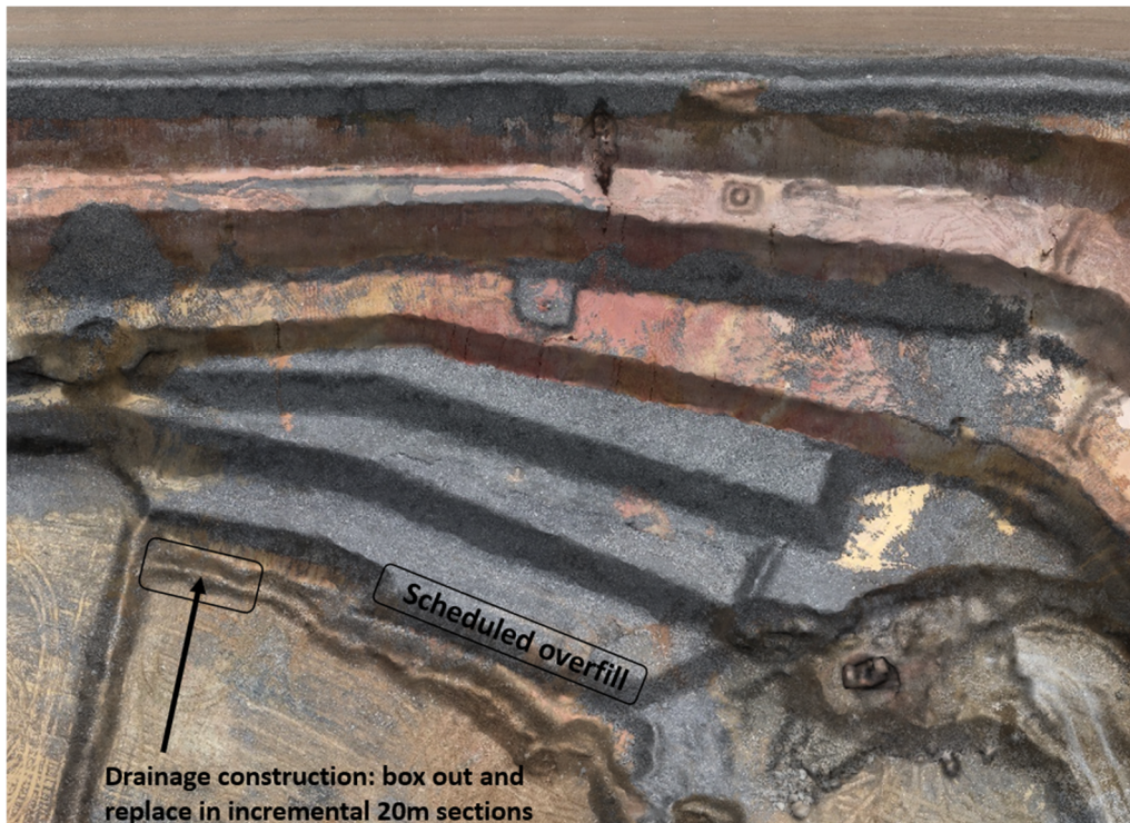
Figure 14 Example of an area to be boxed out and where overfill was placed to promote drainage and stability
