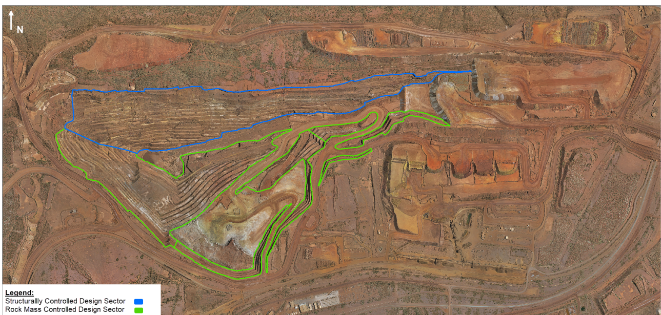
Figure 3 Annotated failure mode area
