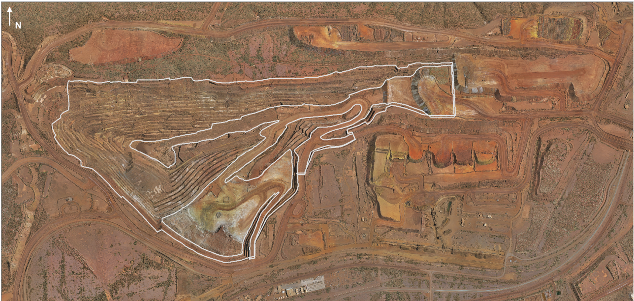
Figure 2 Annotated overall slope area
