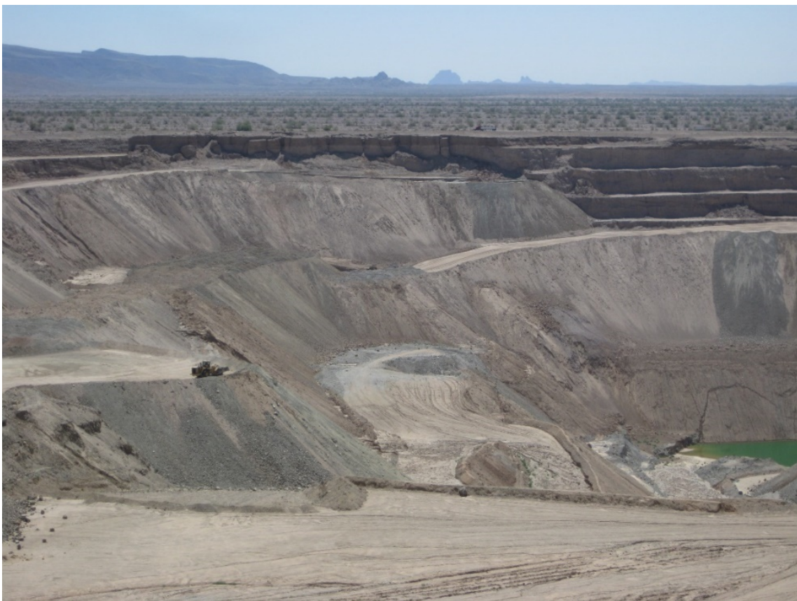
Figure 4 Completed buttress below the east wall of the Rainbow Pit
