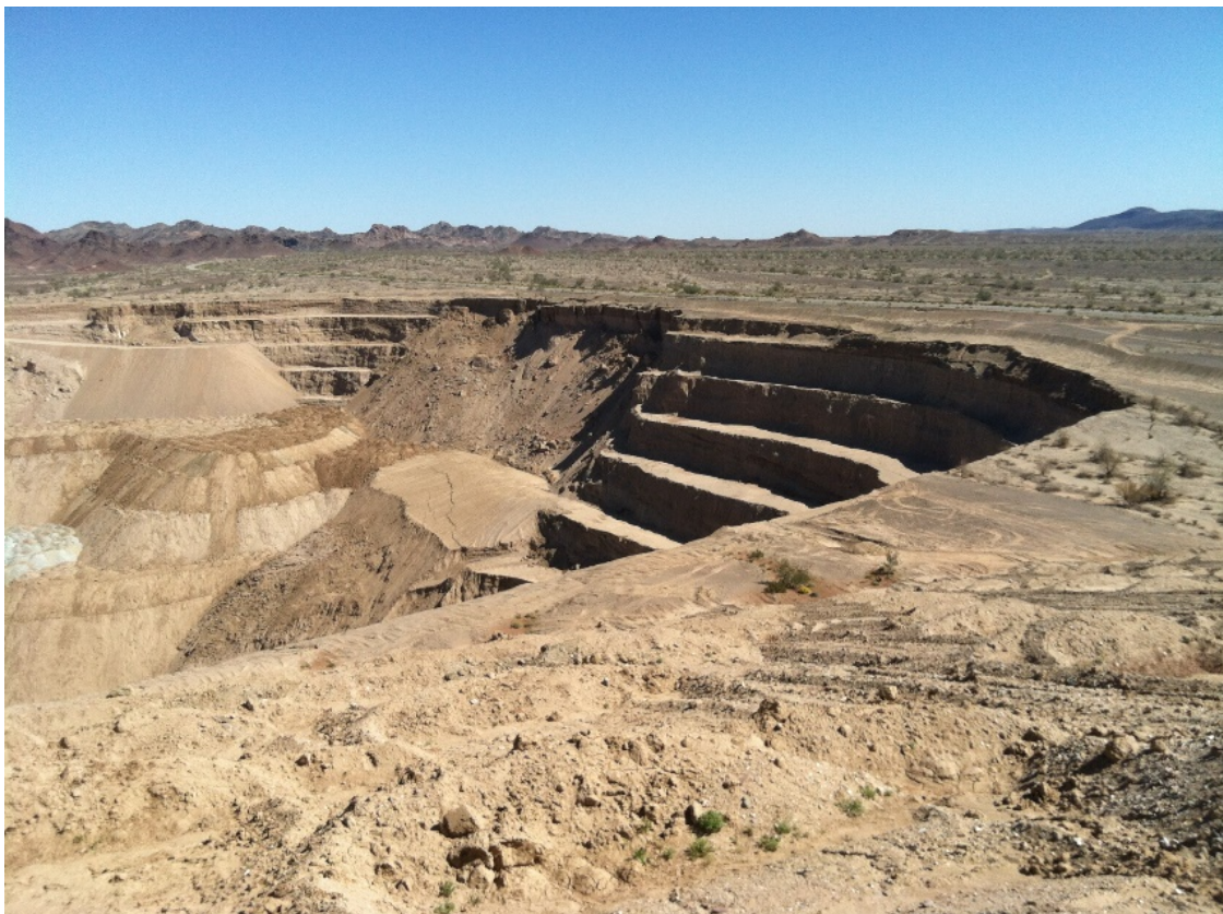
Figure 3 Instability in the tertiary conglomerate gravels materials on the east wall of the Rainbow Pit
