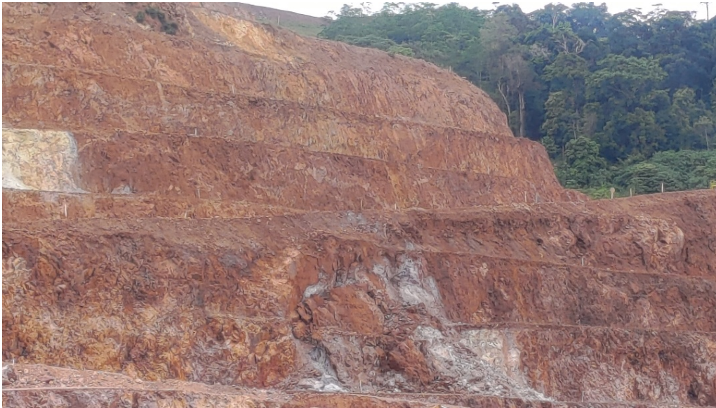
Figure 2 Historical failure of the pit slope
