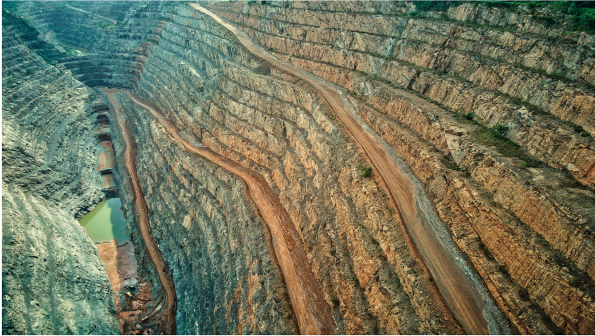
Figure 8 A view of the west wall of the DPCB (camera facing south)
