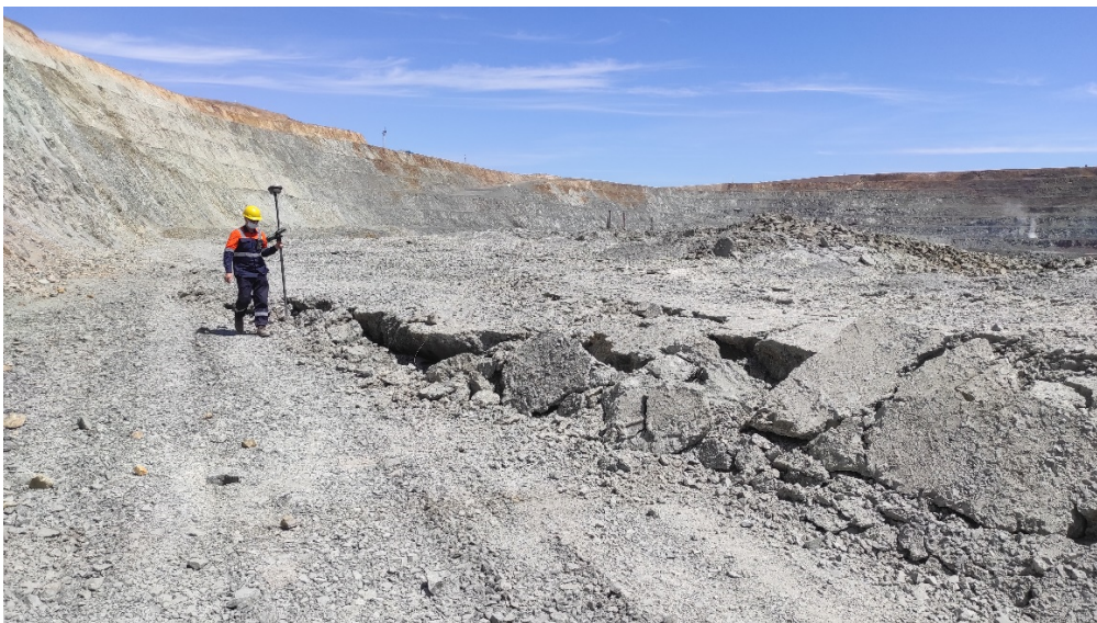
Figure 9 Significant back-break along a fault at Bozshakol pit
