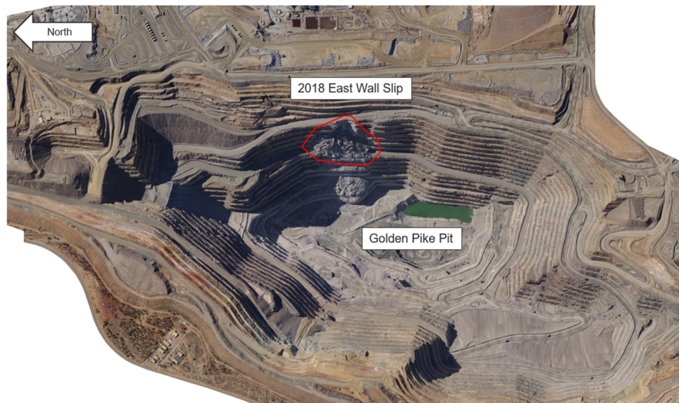
Figure 1 Location of the 2018 East Wall Slip within the KCGM Super Pit (Darbritz 2023)
