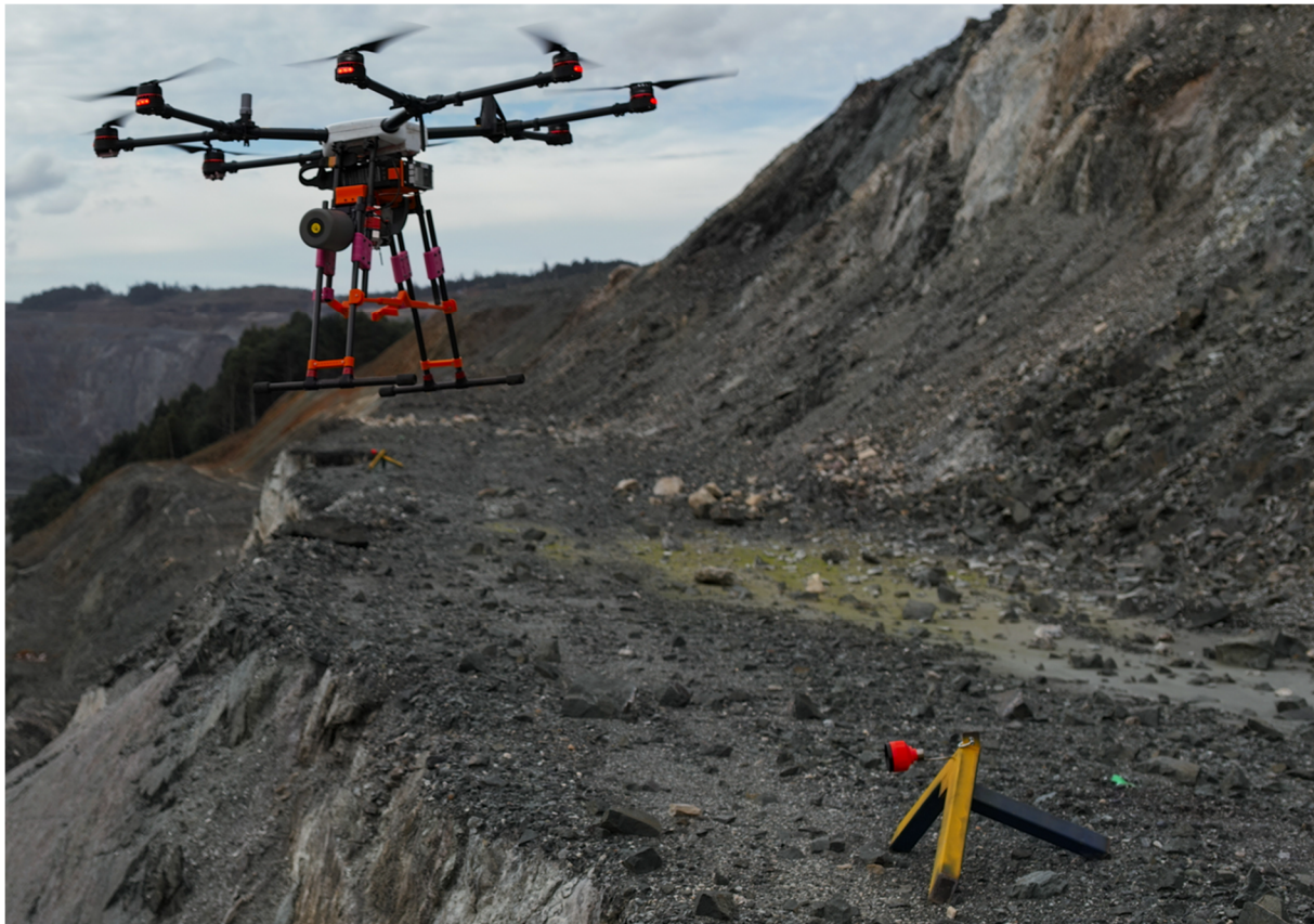
Figure 7 HPRD taking off after dropping a prism in place on a berm
