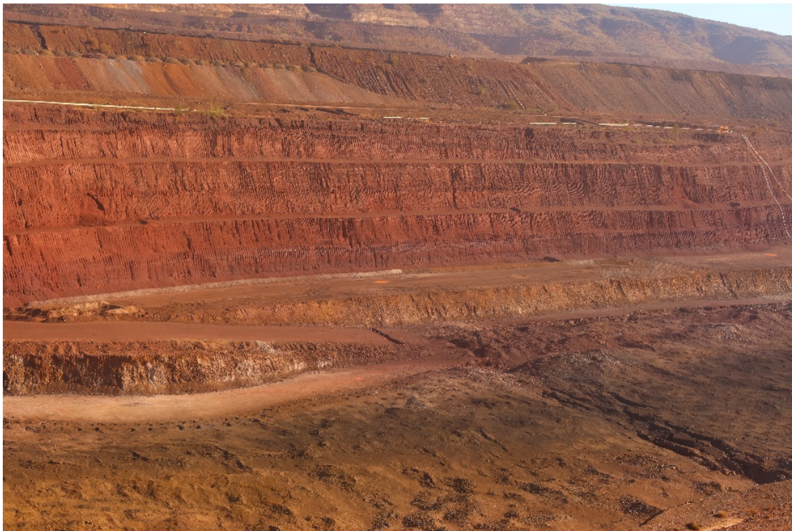
Figure 1 Case study pit slope, prior to deformation and signs of instability
