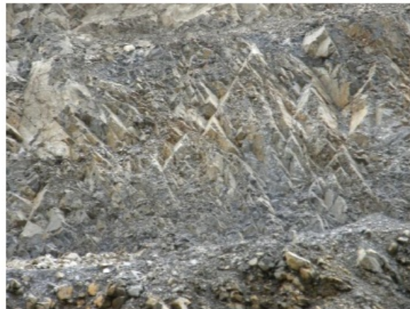
(d) Fresh strong rock, production blasted, fairly effective excavator clean-up of bench face; Ok Tedi, PNG, SE slope (Aug 2011)
