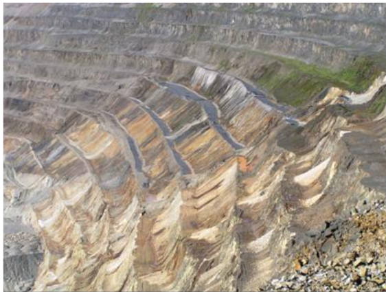
(a) Black HDPE lined bench berm, erosion on unlined berms, Ok Tedi, PNG (Sep 2003)
