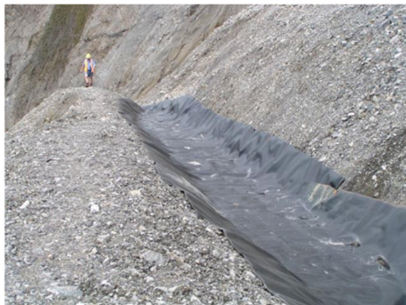
(b) HDPE lined, rockfill-shaped, water drain, Berlin area, West Wall (Mar 2005)
