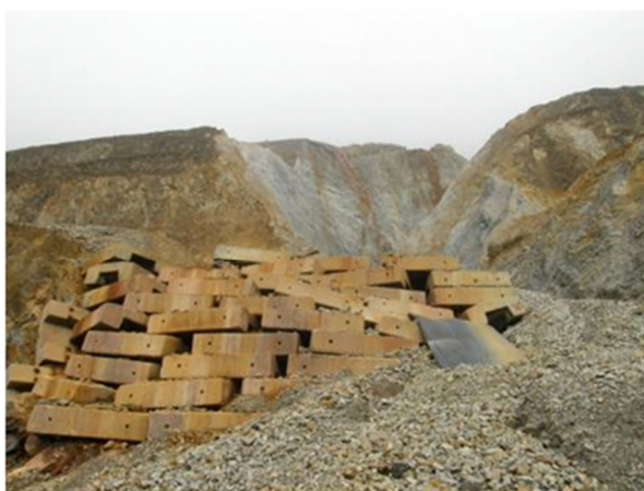
(f) Chasm's V-notch toe buttressed with left-over concrete sleepers from mine's 4km long drainage tunnel, Berlin Chasm (May 2010)
