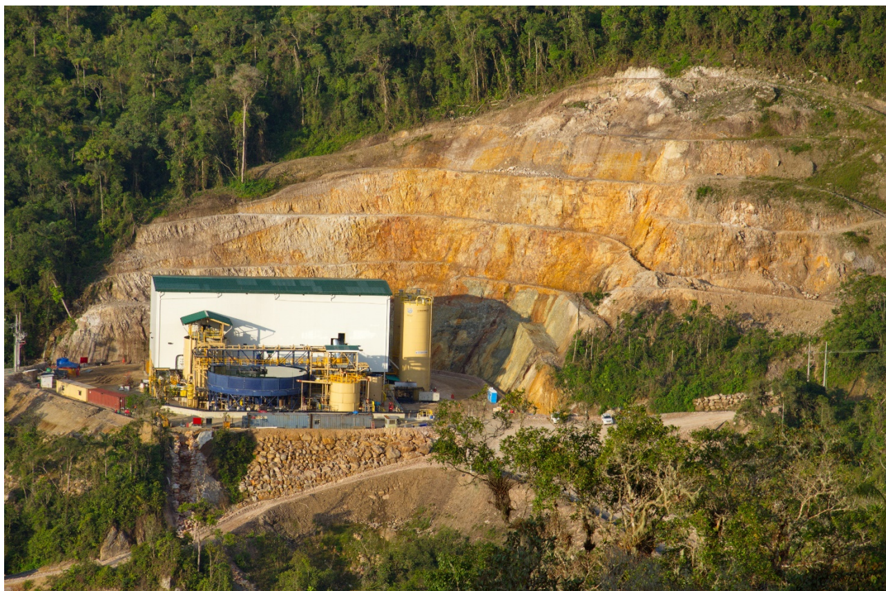
Figure 3 Photo of paste plant showing extent of cut made to create the paste plant platform area
