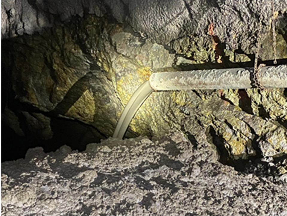
Figure 12 First cemented paste pour at FDN
