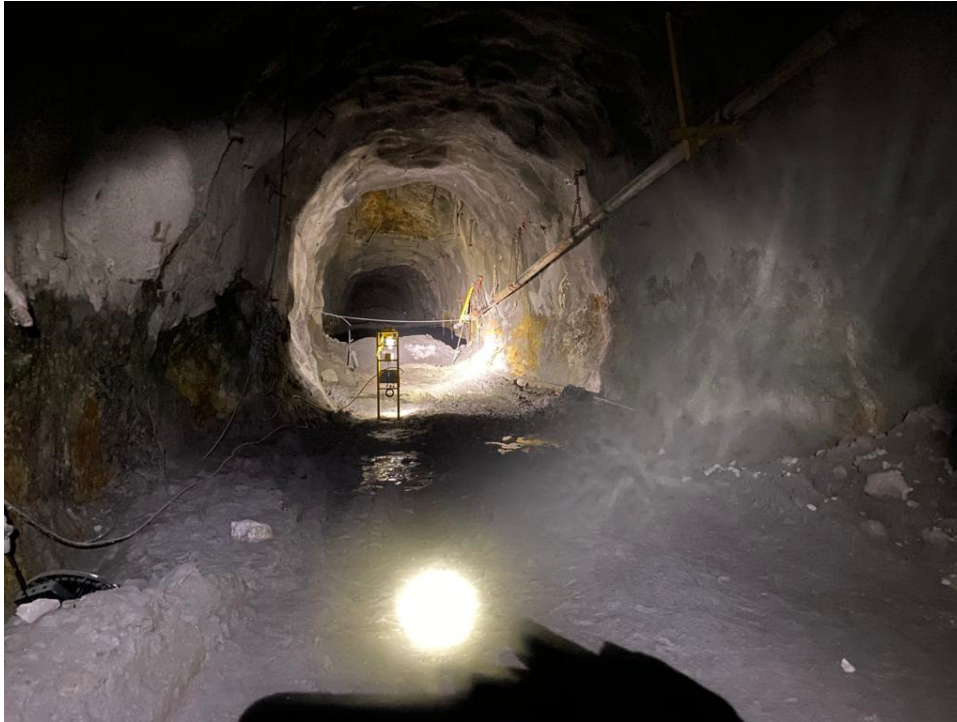
Figure 18 Sending paste to a test stope with berm during commissioning
