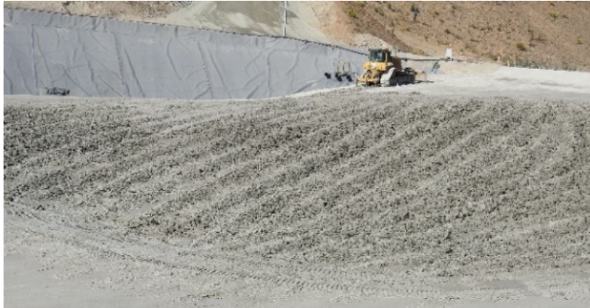
Figure 7 Dozer tilling off specification tailings to allow drying
