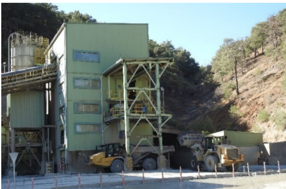
Figure 3 Filtered tailings loading area
