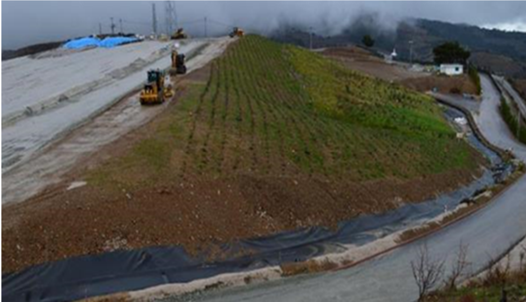
Figure 17 Reclaimed tailings slope following rehabilitation and revegetation activities
