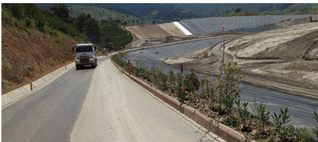
Figure 15 Asphalt paved access road from the filter plant to TSFs
