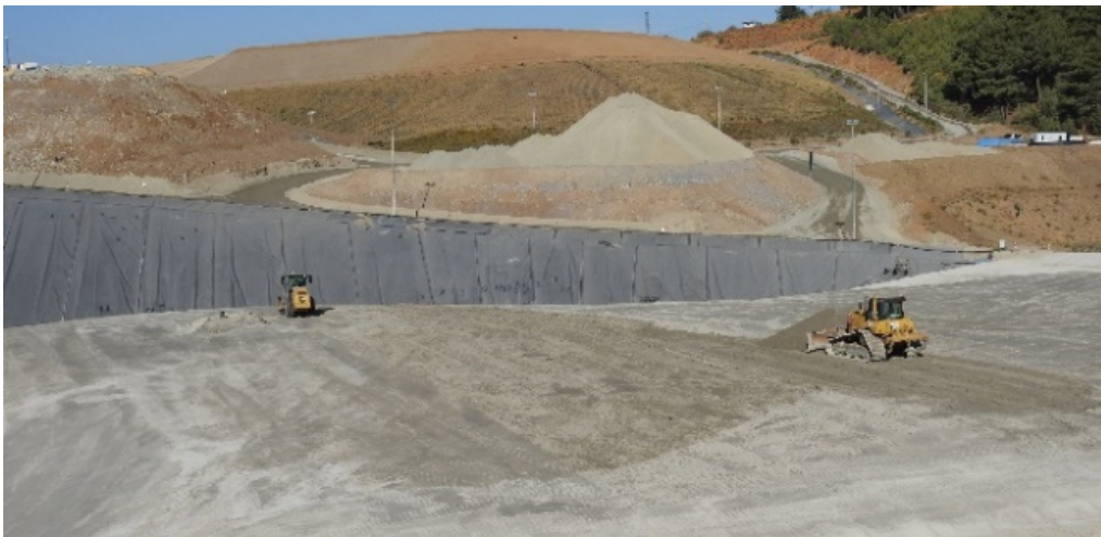
Figure 8 Disturbed area being re-compacted after drying
