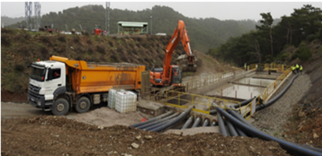
Figure 24 Sediment removal from sediment catchment sump
