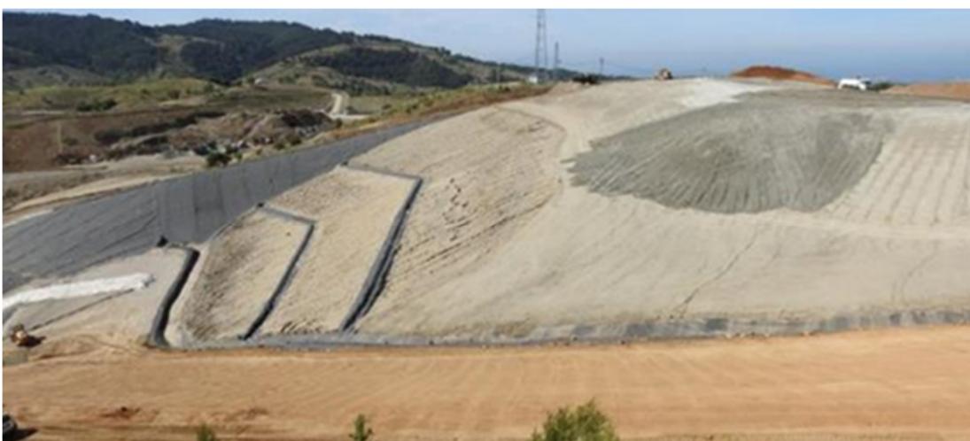
Figure 25 Geomembrane lined channels to reduce erosion and manage runoff
