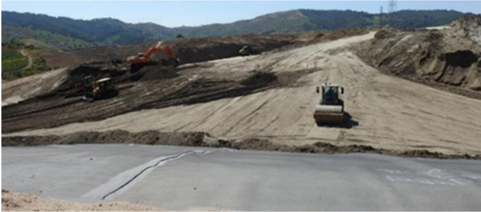
Figure 9 Stockpiled filtered tailings re-handling
