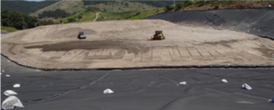
Figure 5 Filtered tailings spreading and compaction
