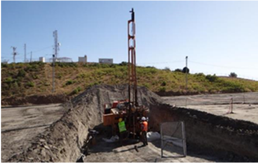
Figure 19 SPT investigation in C-TSF
