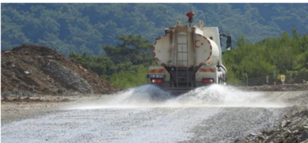
Figure 13 Access and TSF roads are sprayed by water truck
