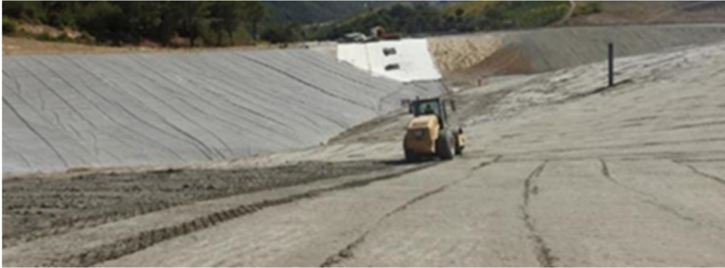
Figure 12 Creating a smooth surficial crust by roller compaction
