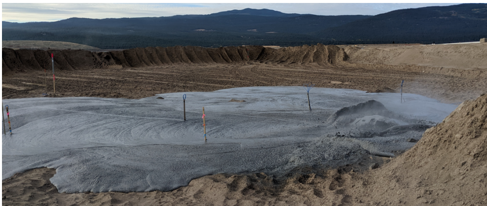
Figure 14 Deposition of thickened and amended tailings to a NATSF test cell
