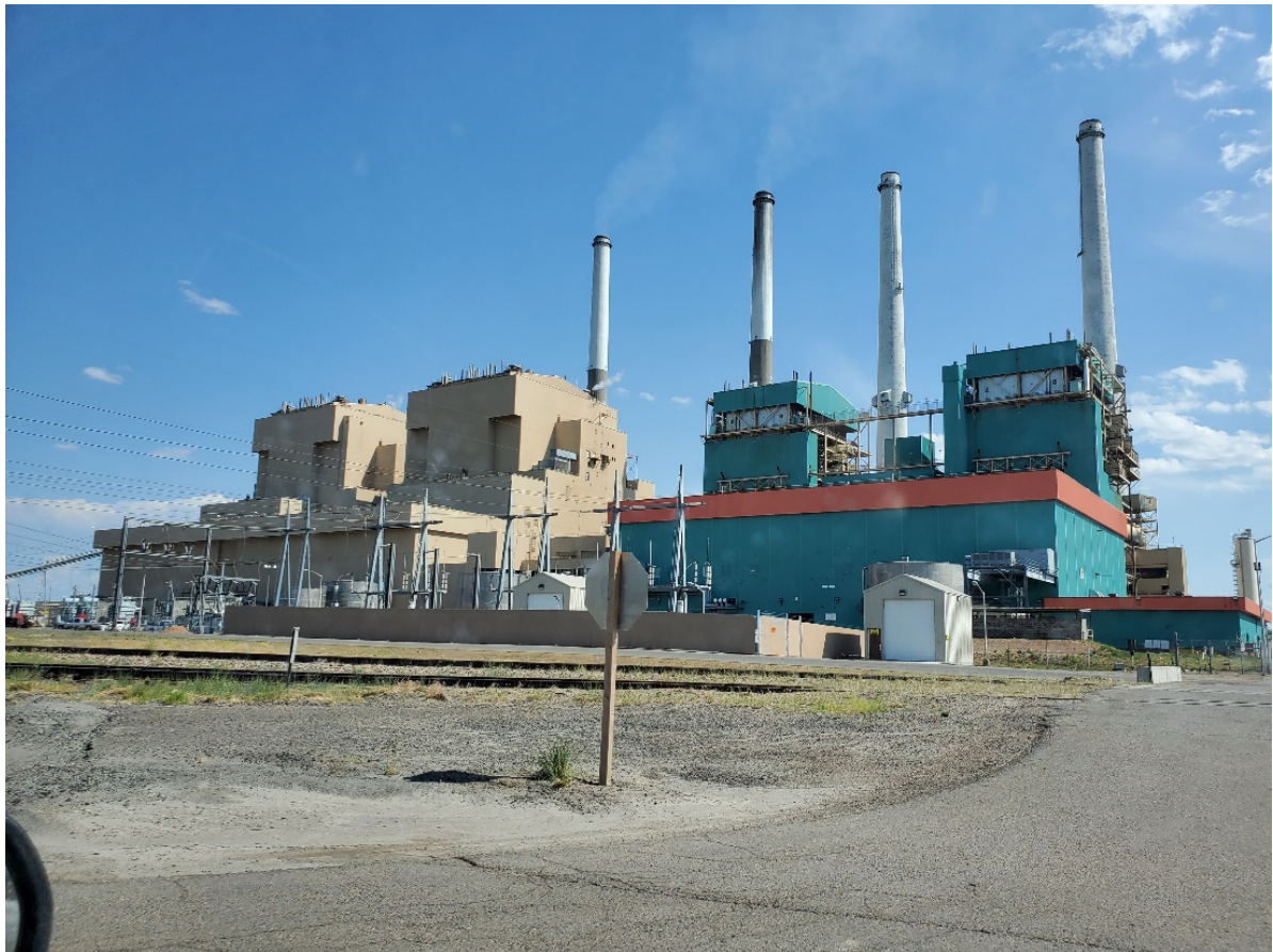
Figure 1 Image of coal power plant with two generators running
