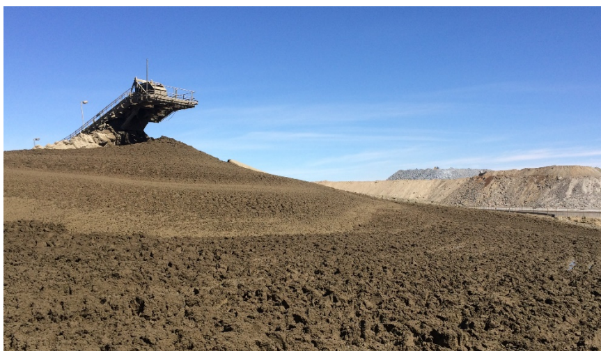
Figure 3 View of the radial stacking system
