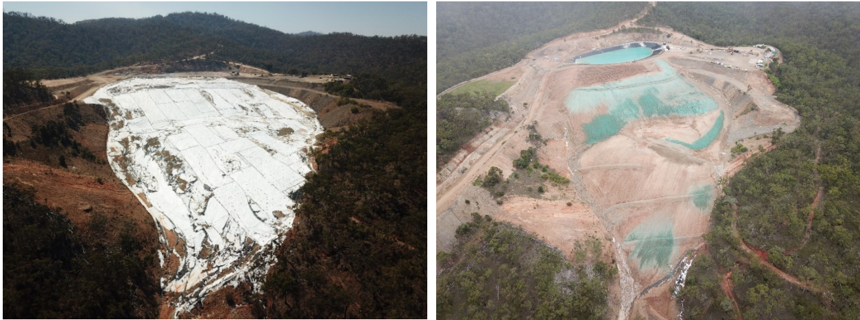
Figure 1 Before and after remediation works on the waste rock dump at Baal Gammon mine
