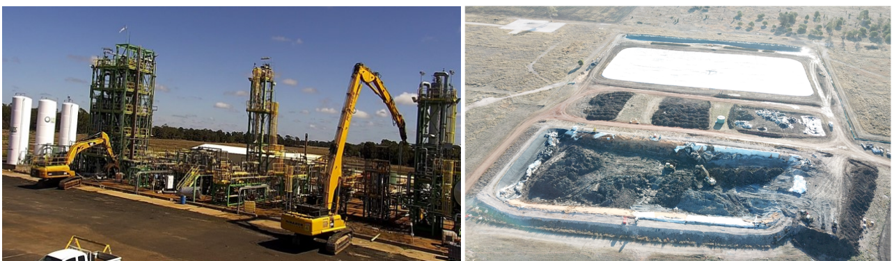
Figure 3 Demolition and remediation works at Hopeland
