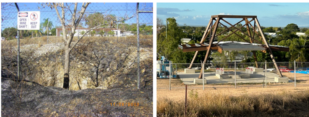
Figure 6 The shaft before and during remediation works in Charters Towers
