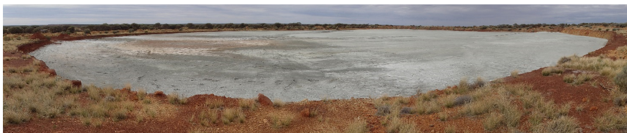
Figure 1 In-pit tailings disposal at the Perch pit (Plutonic mine, Pilbara, Western Australia) (CD McCullough)
