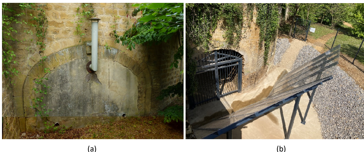
Figure 7 Reopening of an adit closed after mining operations ceased to ease natural drainage of the mine gas: (a) Before reopening in July 2020; (b) After reopening in April 2024, with safety devices (inclined deflectors and fences) to prevent people from being exposed to mine gas emissions (photography by BRGM-DPSM)
