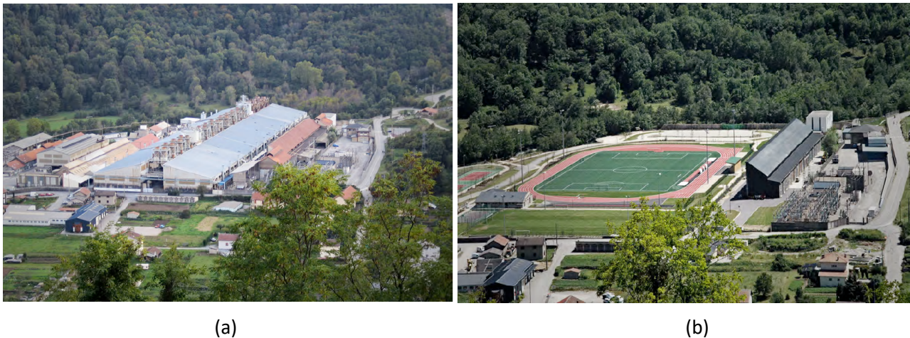
Figure 2 (a) The Auzat aluminium smelter in 1990; (b) The site transformed in 2011
