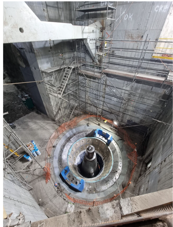
Figure 12 Crusher Chamber Construction
