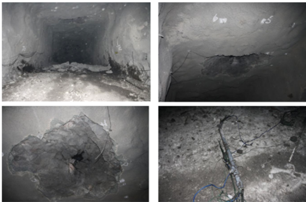
Figure 12 Spall damage due to reflection mechanisms when primer location was 8m from the top of the stemming zone.
