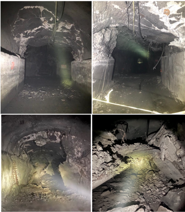
Figure 9 Sequence of damage observed in the extraction throughout the collapse process.
