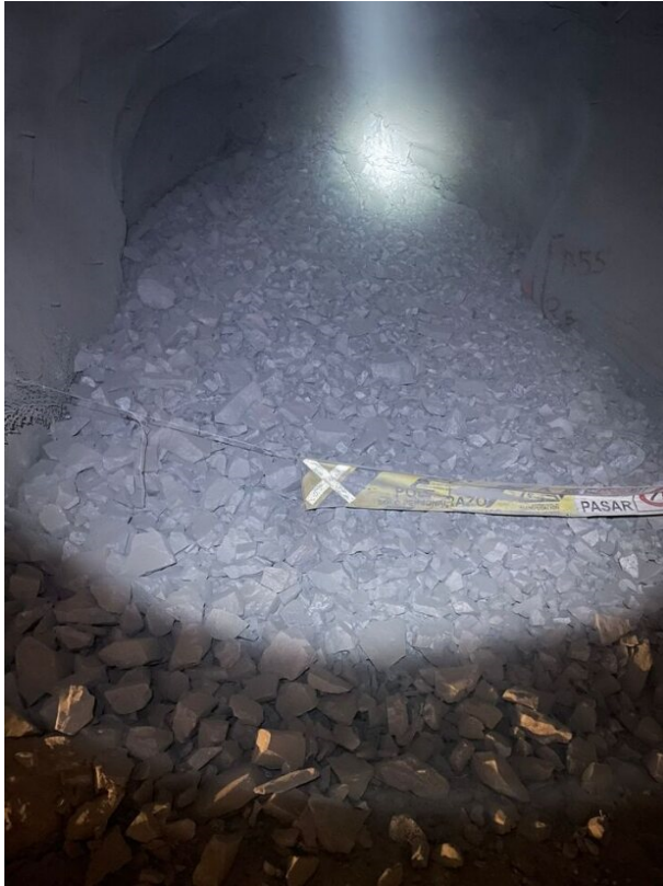
Figure 26 Post-blasting fragmentation pile.
