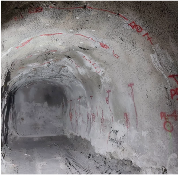
Figure 21 Marking and cleaning drillholes.
