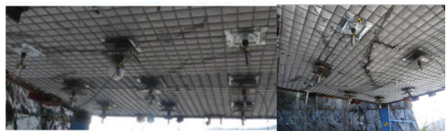
Figure 23 Ground Support System S-B3: Pre and Post Impact Test Configuration.
