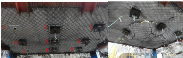
Figure 25 Ground Support System S-B4: Pre and Post Impact Test Configuration.
