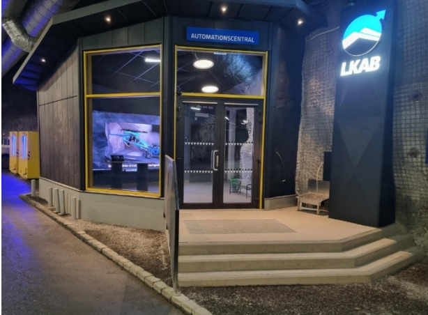
Figure 8 “Control room of the future” built to handle all Autonomous applications, located at the 1250m level in Malmberget Mine.
