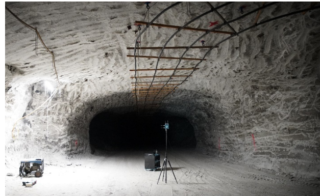
Figure 3 Final installation of the radiating cables in the drift.
