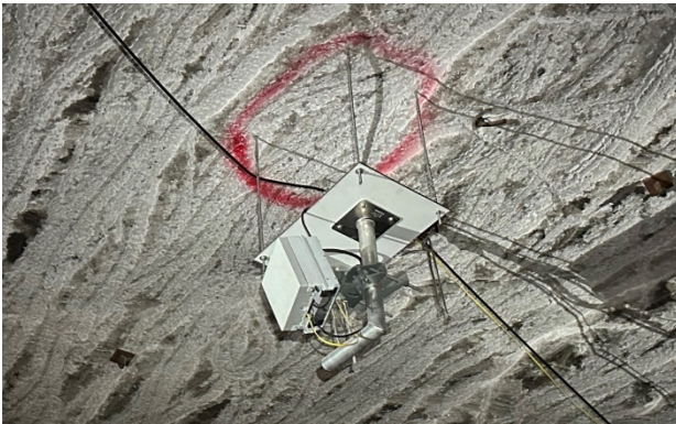
Figure 2 Final installation of the directional radio (Ericsson 4408) in the mine workings.
