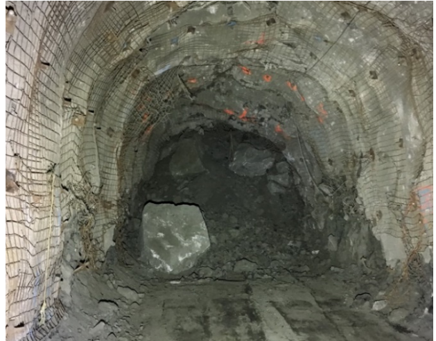
Figure 13 Granite wallrock oversize dilution in an A418 drawpoint.
