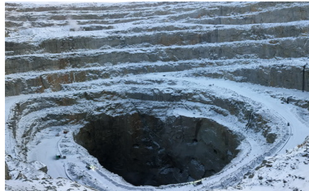
Figure 9 Empty SLR stope at the bottom of the A154 Open Pit.
