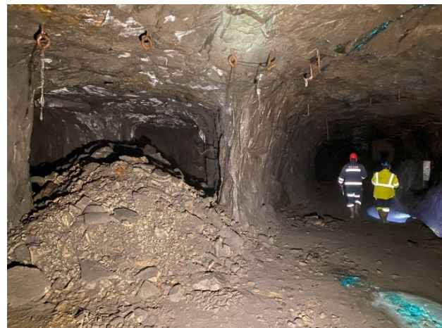
Figure 5 Footwall drift (right) and extraction drifts (left) on Kapten level 460 m.
