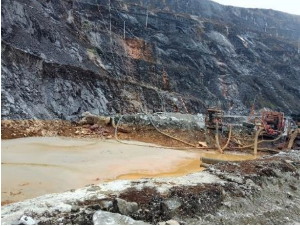
Figure 7 Grasberg sump and pump condition.
