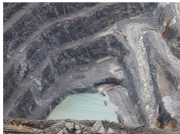
Figure 14 The condition of Grasberg bottom pit with amole drift during the storm event.
