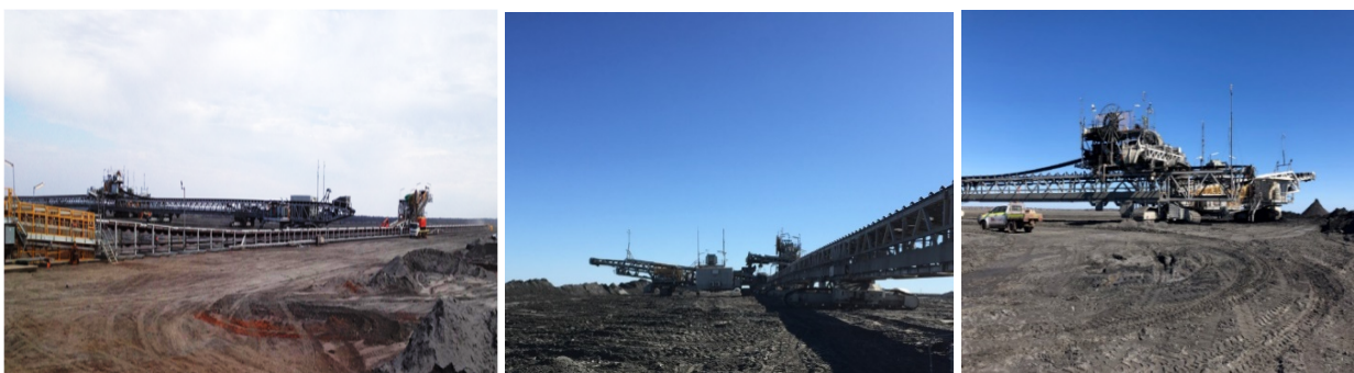
Figure 19 Mechanical conveying and stacking equipment for FTSF (equipment-intensive operation)
