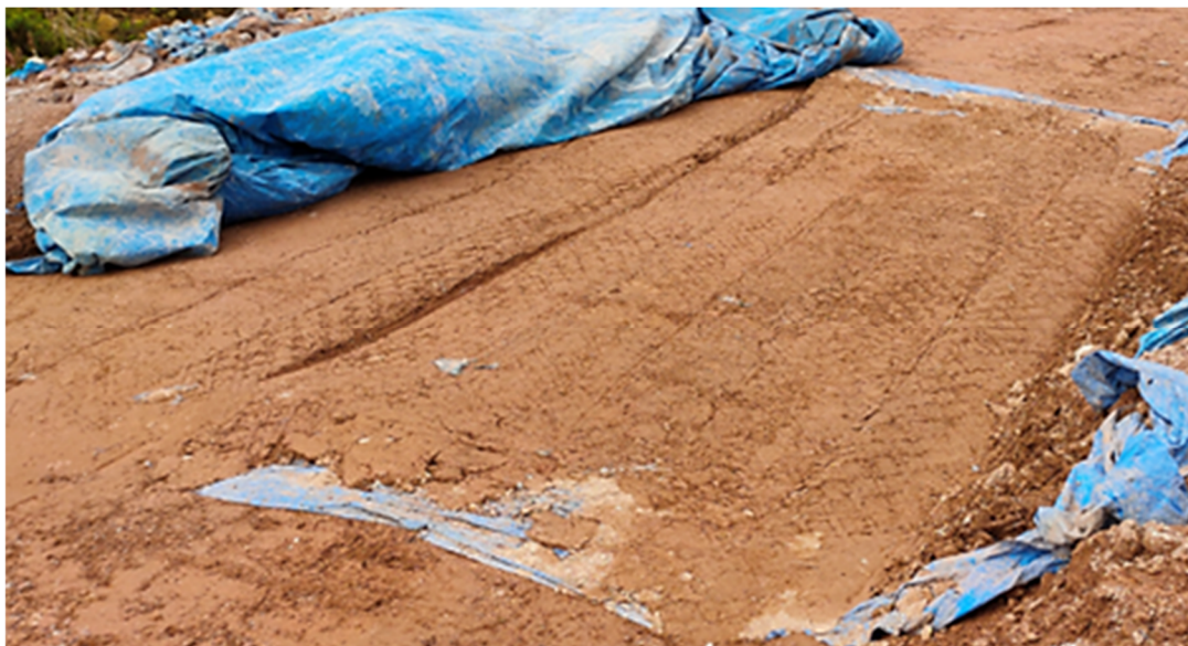
Figure 15 Compacted co-disposal during field trial
