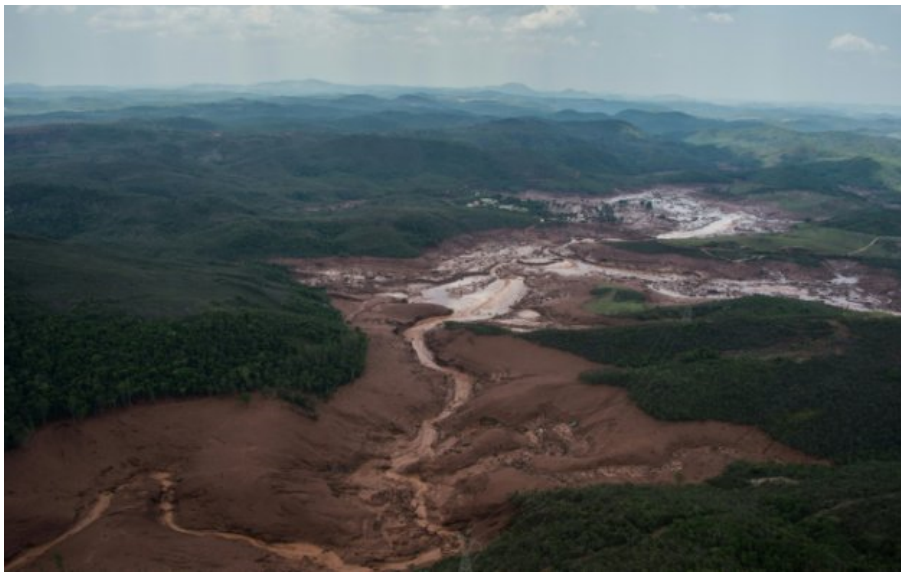
Figure 3 Feijão dam's collapse 2019
