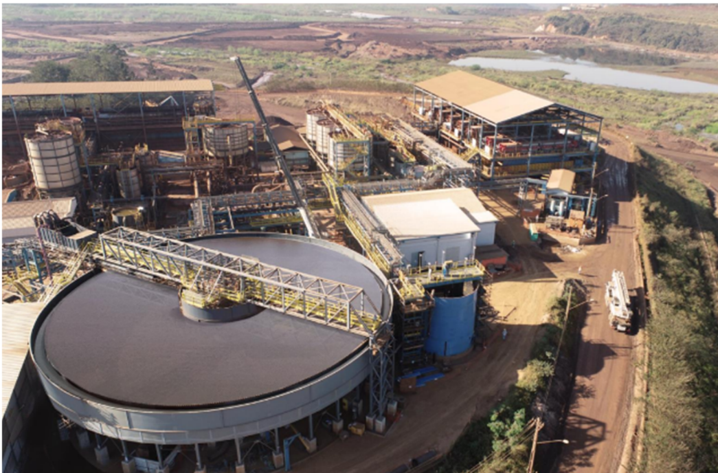
Figure 9 Companhia Siderurgica Nacional plant completed with the final expansion
