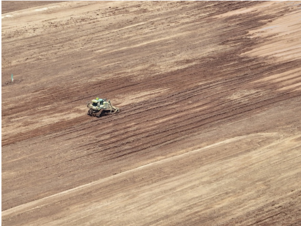
Figure 11 Compaction of tailings, also known as mud farming, being undertaken with a low-ground pressure undercarriage dozer at a tailings storage facility in Australia
