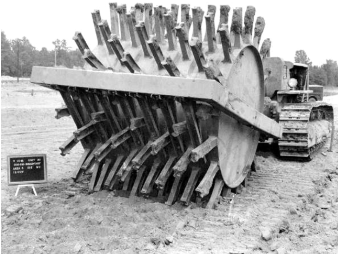
Figure 2 Modified Proctor roller
