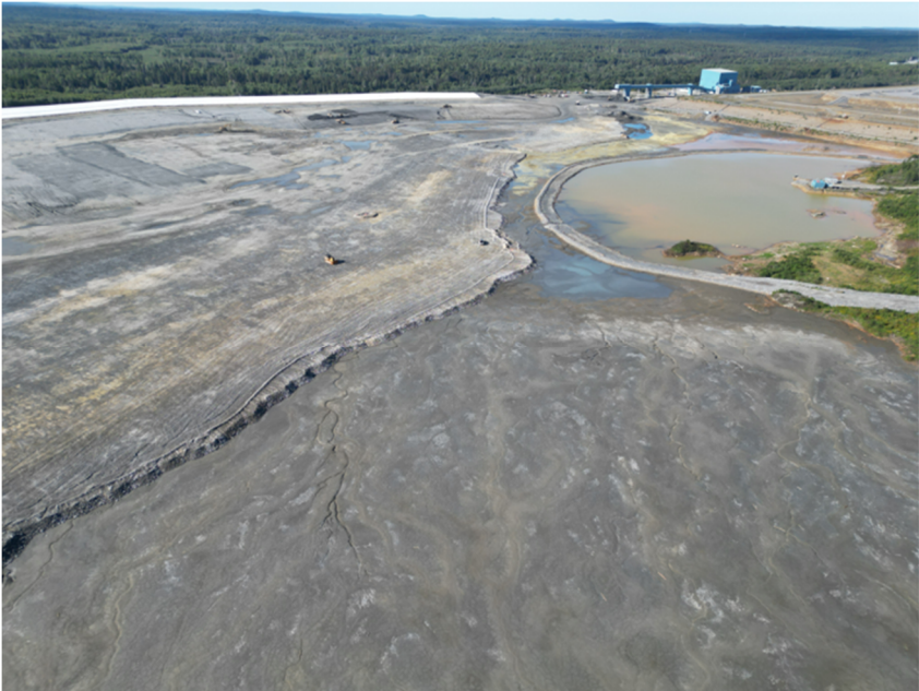
Figure 3 Bridgelift construction over Extension A4 TSF (September 2023)
