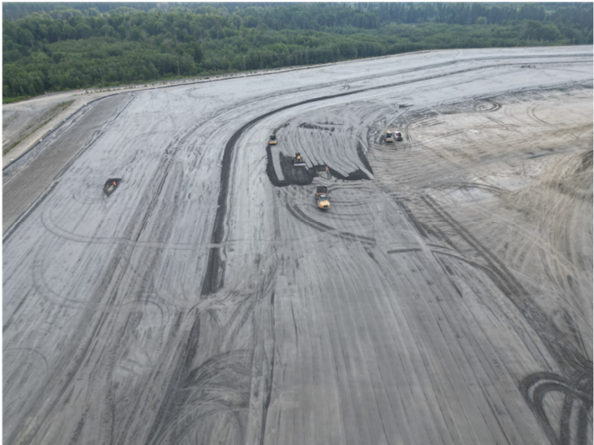
Figure 4 Filtered tailings stack construction (September 2023)
