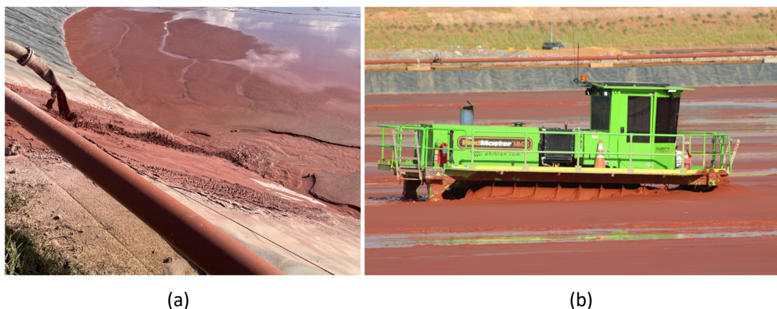
Figure 2 (a) Active discharge of tailings into TSF A; (b) MudMaster conducting AMC recovery work on TSF A
