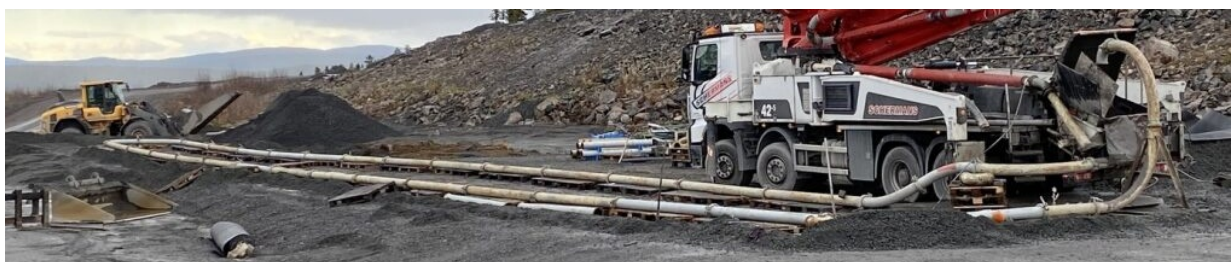
Figure 2 Loop test set up with a 94 m long steel pipeline with smooth bends
