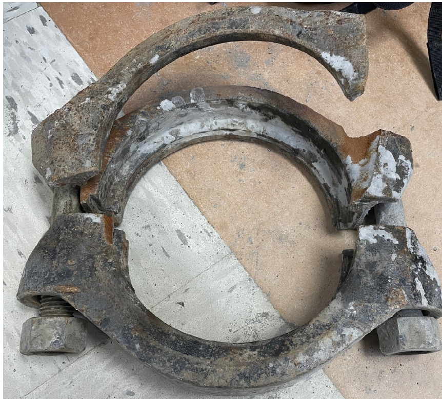
Figure 13 Backfill pipeline coupling failure from fatigue loading
